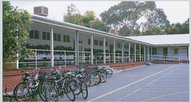
6 units installed at Coolbinia Primary School, Perth Western Australia.
